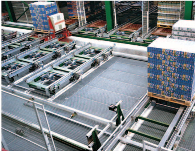
EISENMANN automated warehouse in Morbegno, Sondrio
