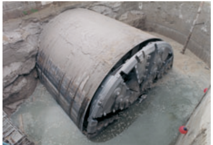
Tunneling machine finishing the fourth bore
