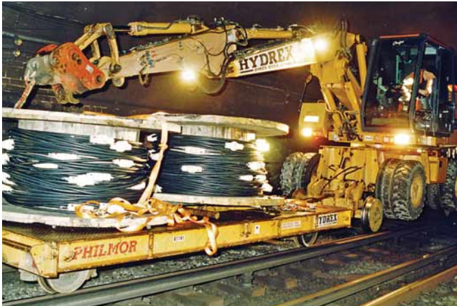
Underground emergency lighting installation
