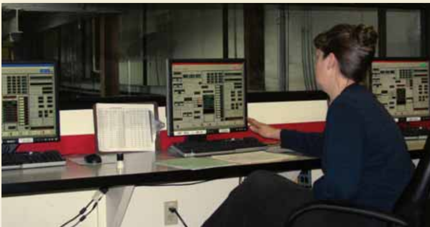
Figure 1: Bodycote control room.
