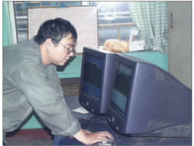
Operation and control room
