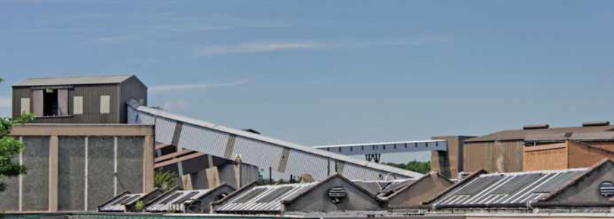
Daw Mill Drift Mine Conveyors
