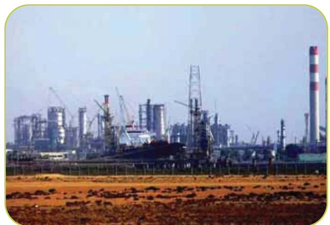
The Invensys solution covers the entire refinery and petrochemical complex comprising 23 plants.
