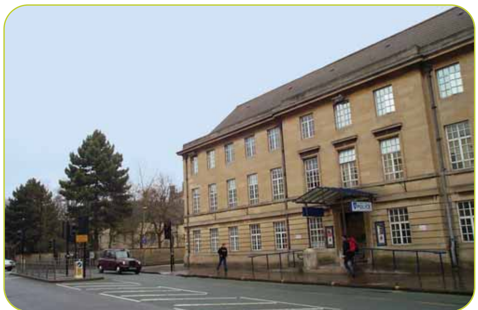
Savings are possible in any building regardless of size age or usage.
